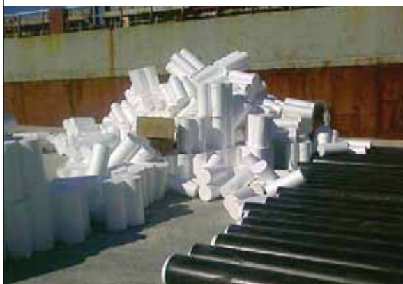
PLATE 40 Polystyrene cylinders are inserted into the pipes
