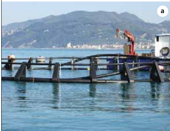
PLATE 39 Sinker tube. a) the sinker tube is temporarily fastened onto the cage handrail, to facilitate transportation from the harbour to the site; b) an installed sinker tube
